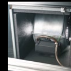
Motor box with soundproofing panels
